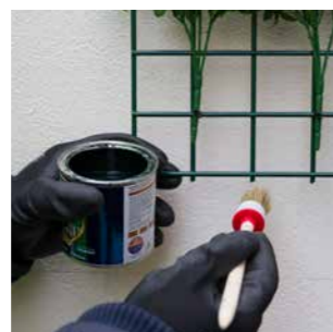
STEP 4 Protect cut point with metal paint.
