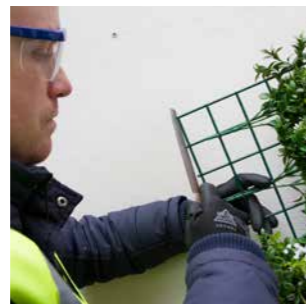
STEP 3 File the grid after cutting.
