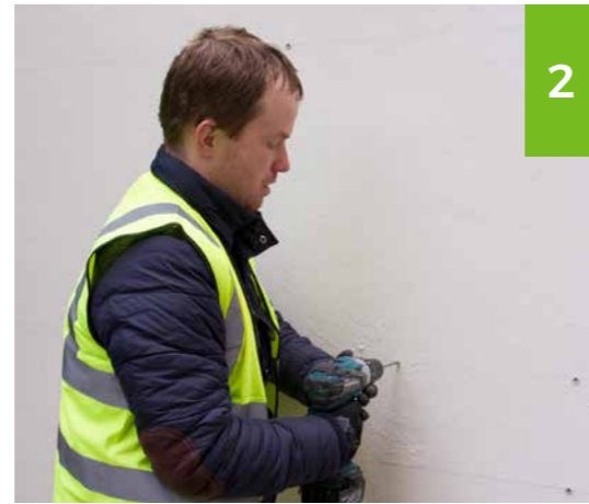
Drill the holes
