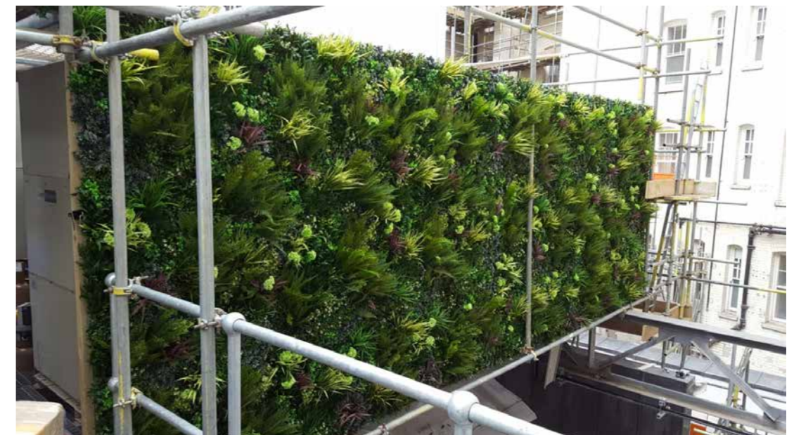
Completed project dressed with Delicate White Colour Box prior to install due to complicated access to the wall
