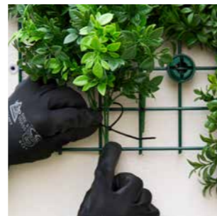
STEP 5 Re-attach loose plants from the vertical off-cuts with cable ties.
