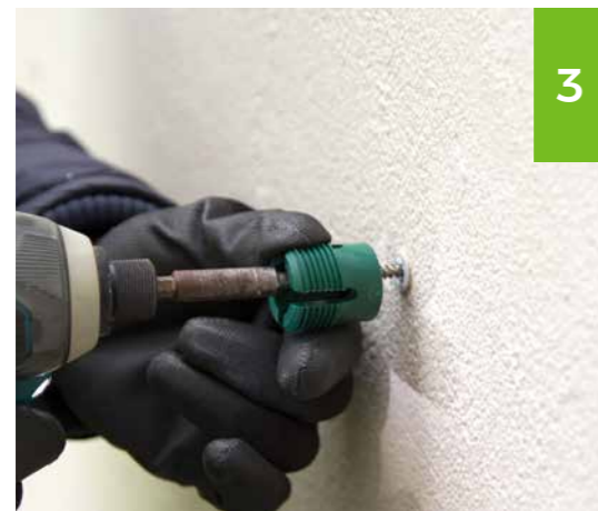
Plug & screw the fixing
