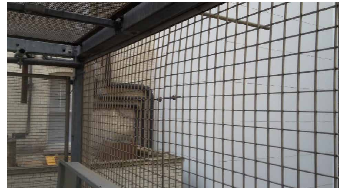
Metal cage before Vistafolia® Panel installation
