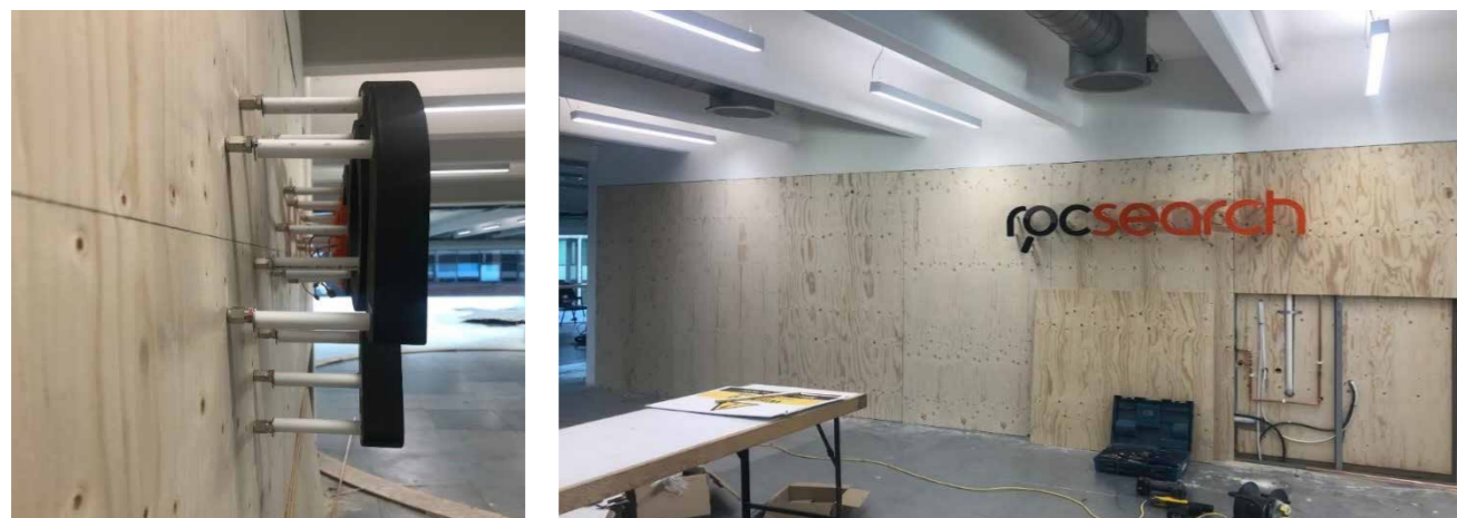
Fixings of the sign – letters to be removed before panel installation
